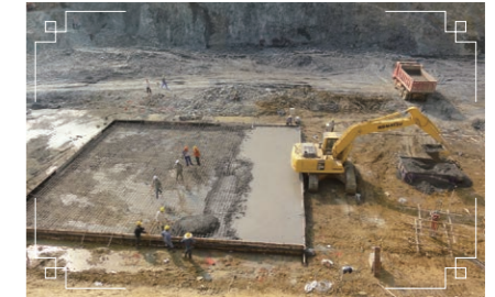
Capital construction site of the Xiaohei River Huilong Mountain Hydropower Station.
