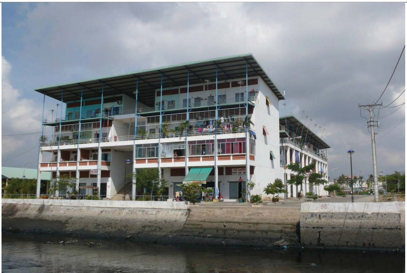
D. 6, W.11 - Apartments along Tan Hoa Lo Gom canal
