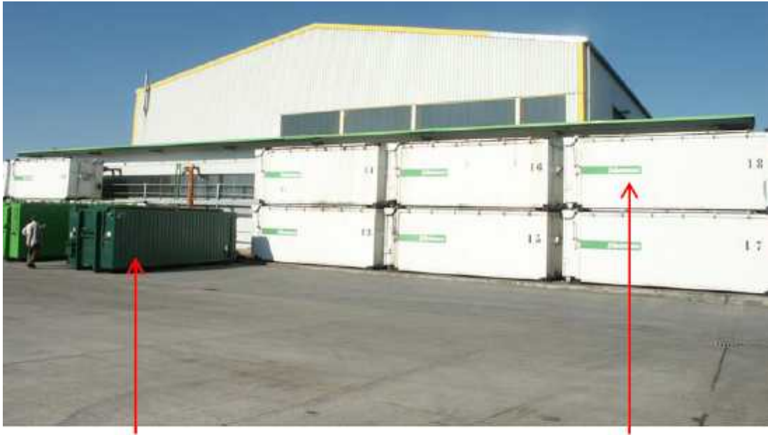
Newer container design attached to the process
